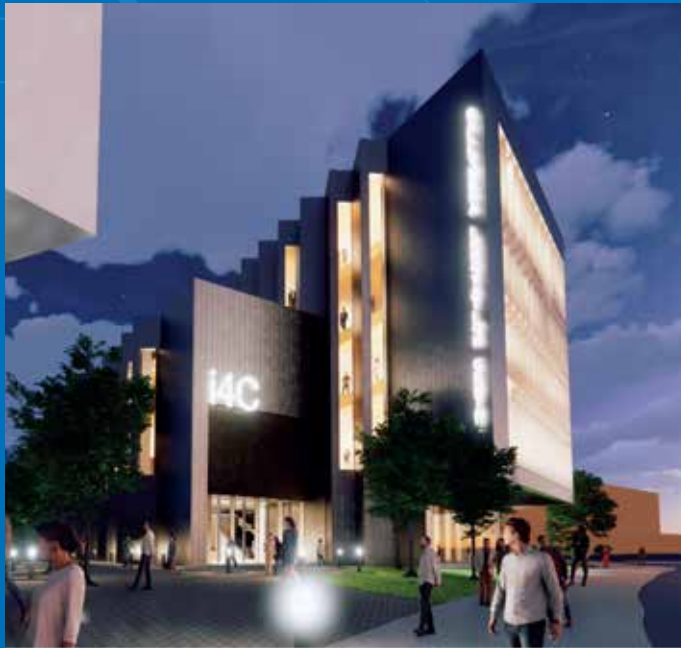
The south facing façade would have a series of industrial style jigsaw window openings to prevent overheating and to prevent the building overlooking new residential housing developed by Radius. The siting and building mass of the new NRC campus can be seen in the background.
